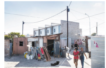
Figure 88: Site selection identification and emphasis through the engagement of the Empower Shack project in Khayelitsha, Cape Town. Source: Urban-Think Tank, Alfredo Brillembourg & Hubert Klumpner, http://u-tt.com/project/empower-shack/ ; accessed 13.02.2021
