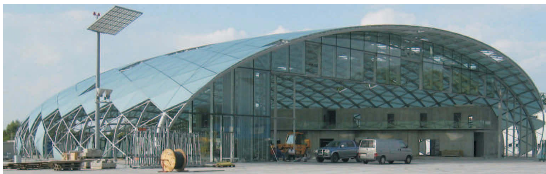
Figure 8. Double curved surfaces like ellipsoids can only be triangulated or produced by cutters, unless made of concrete. No matter how careful or cunning the triangulation is, as with this ellipsoid “Hangar 8” by Volkmar Burgstaller (©Metallbau Pagitz, reprinted with permission), there two major drawbacks that cannot be overcome: First, it is impossible to do so in a way that all triangles are equally shaped. Second, the surface will never look entirely smooth.
