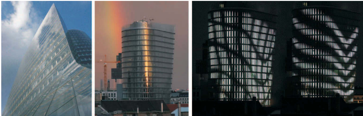
Figure 16. Heinz Neumann, Uniqa Tower Vienna (photos G. Glaeser). Straight contours immediately help to detect a torsal surface. At night, the surface is visually changed by light effects
