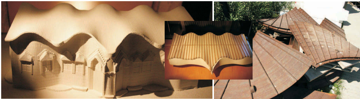
Figure 25. A. Gaudi’s proposal for the construction of “almost” developable ruled surfaces (exhibited in Casa Milà, Barcelona, photos G. Glaeser): Chose the middle line and rotate rods intersecting perpendicularly. The results are conoid surfaces [5]
