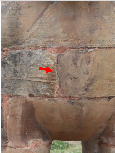
Fig. 1: Thin joint section open.
