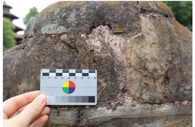
Fig. 4: Microbiological growth and lichen on the top part.
