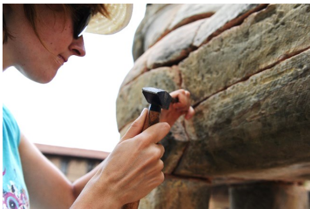
Fig. 3: Removal of former joints, 2011
