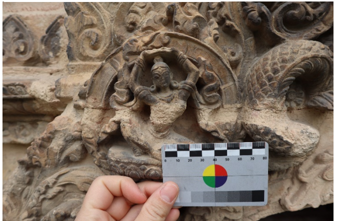
Fig. 4: Joints cracked along the edges to the stone.
