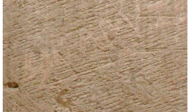
Fig. 4: Detail of fine processing with chisel
