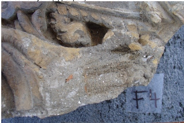
Fig. 14: Detail of thin cement coating on the surface
