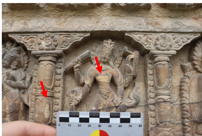
Fig. 5: Scaling on stone surface.
