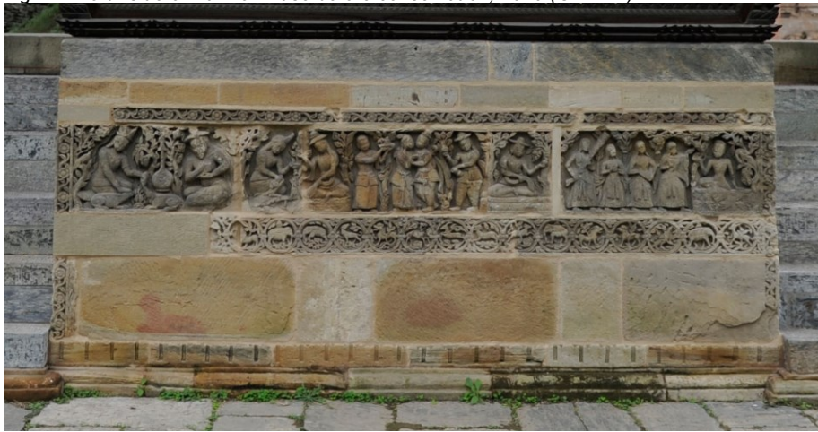
Fig. 23: North side of Pavilion Base after conservation, 2014
