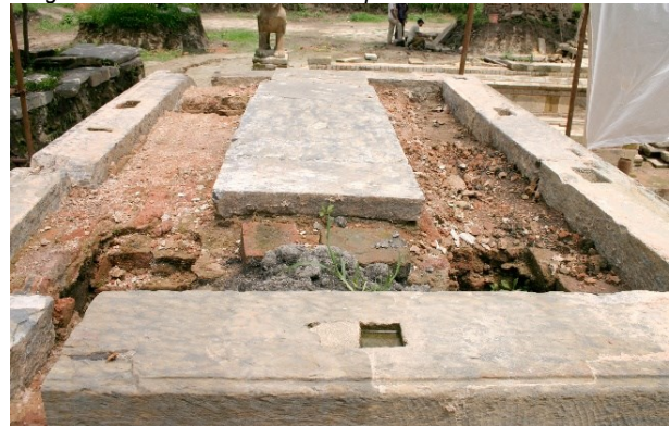
Fig. 11: Mud on top of seating, calcitic schist capping/frame
