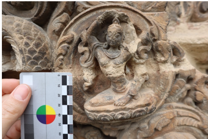
Fig. 3: Joints cracked along the edges to the stone.
