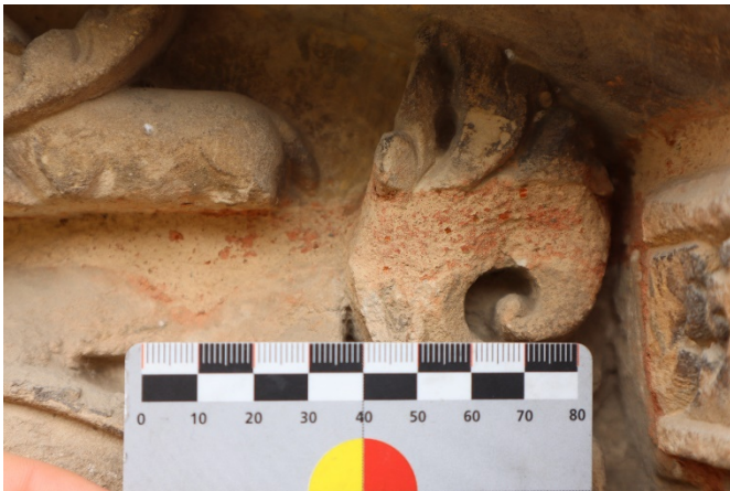
Fig. 8: Powdering of joint retouching.
