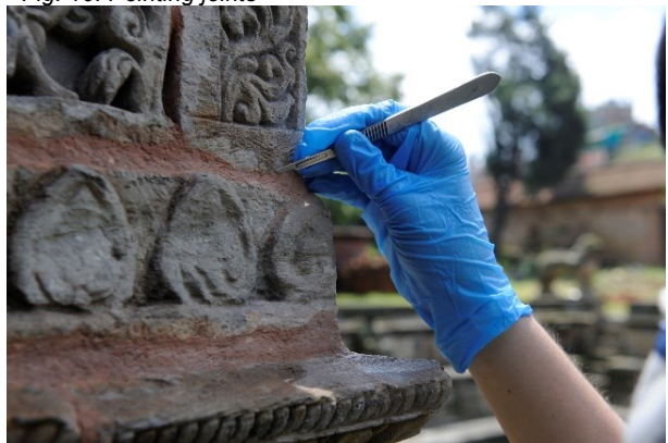
Fig. 21: Reducing mortar residues
