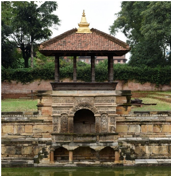
Fig. 1: Overview of pavilion facing the tank, 2014
