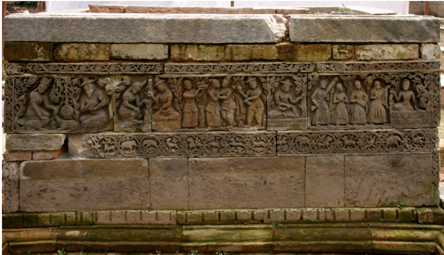
Fig. 22: North side of Pavilion Base before conservation, 2010 (© KVPT)
