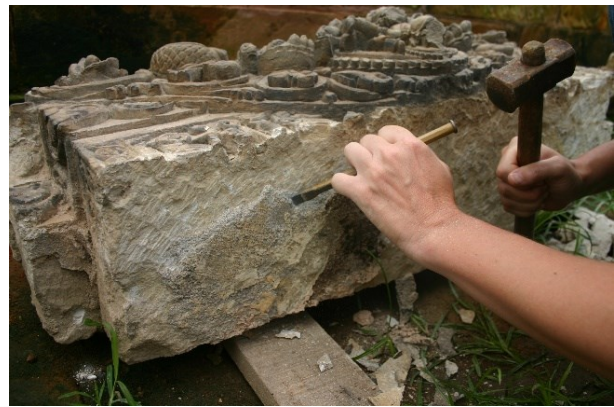
Fig. 17: Removing former (cement) mortar
