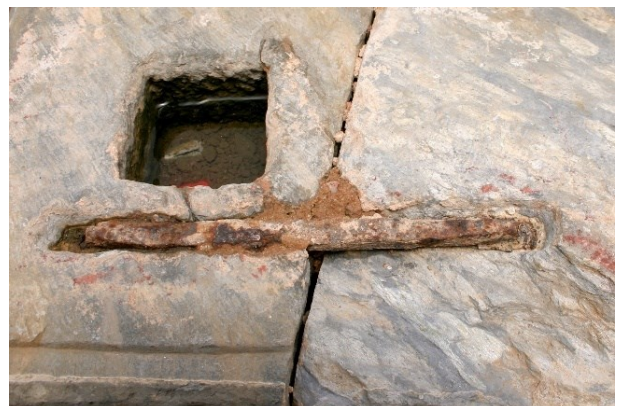
Fig. 9: Detail of former iron clamps
