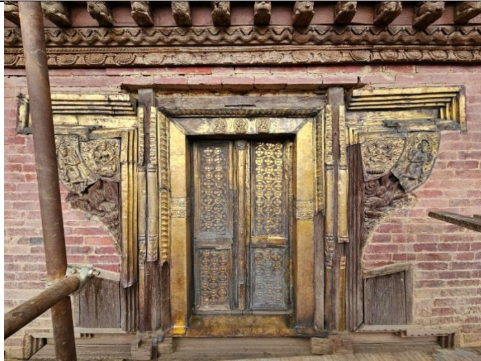
Fig. 1: Golden door on the fourth floor after cleaning, 2023
