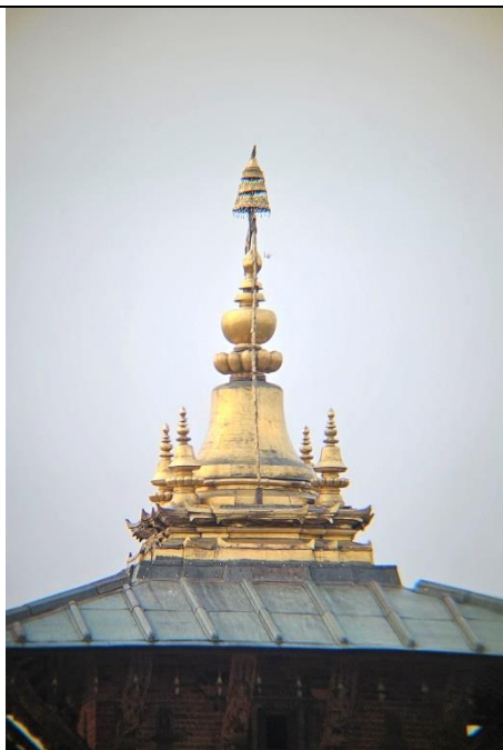
Fig. 15: Finial and roof, S-side, May 2024
