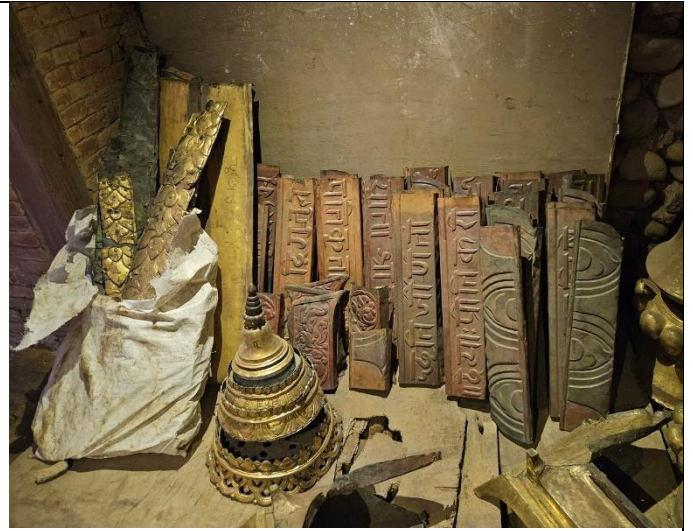
Fig. 8: Copper sheets, top piece and repoussé decoration of the roof after conservation, 2022
