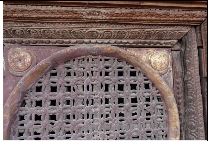
Fig. 21: Window covered in dust from construction work, May 2024
