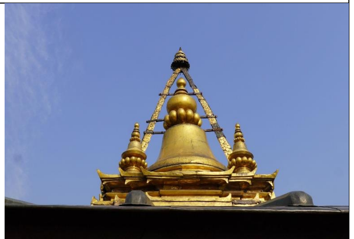
Fig. 12: Pinnacles and base assembled, E-side, May 2024
