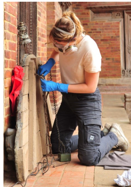
Fig. 18: Polishing the surface
