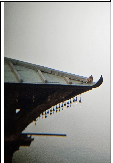
Fig. 17: Roof edge, May 2024
