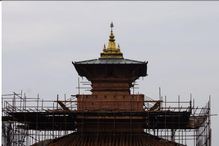
Fig. 13: Finial and roof sheets assembled, N-side, May 2024
