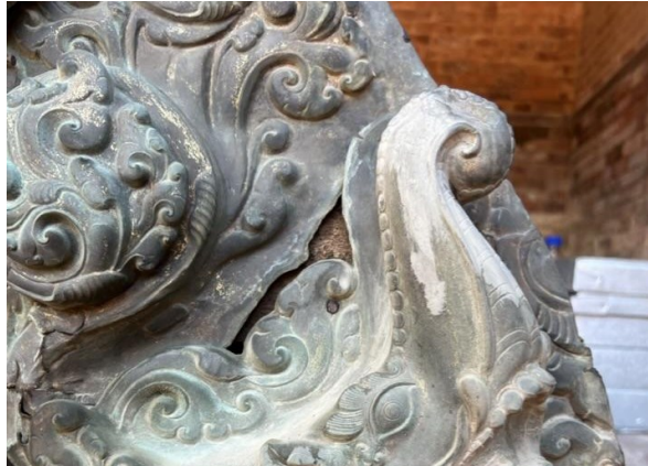
Fig. 12: Surface covered with dirt
