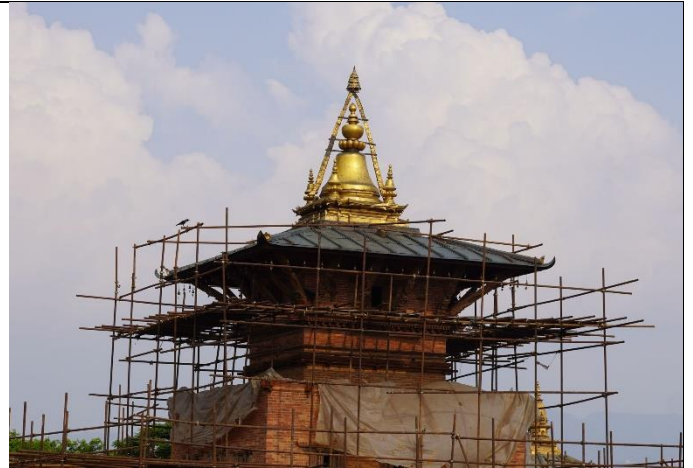
Fig. 14: Finial and roof sheets assembled, W-side, May 2024
