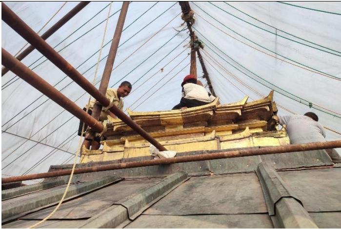
Fig. 9: Assembly of the kulām and mikhāphusi base of the pinnacles, May 2024 (© Bikash)
