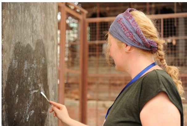
Fig. 16: Mechanical cleaning of stone
