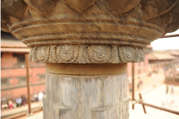
Fig. 5: Metal ring at the column shaft
