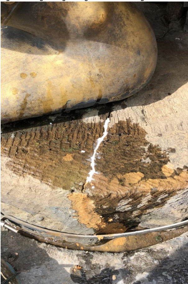
Fig. 22: Filling of crack in plinth with mortar
