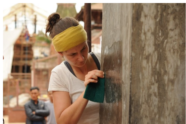
Fig. 17: Mechanical cleaning with non-woven web
