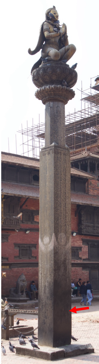
Fig. 2: Darkened area due to oil and other greasy substances.
