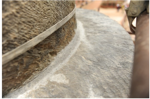
Fig. 19: Derusted metal ring, pointed joint
