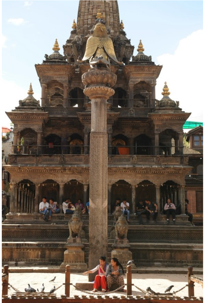
Fig. 24: Overview after conservation, 2018
