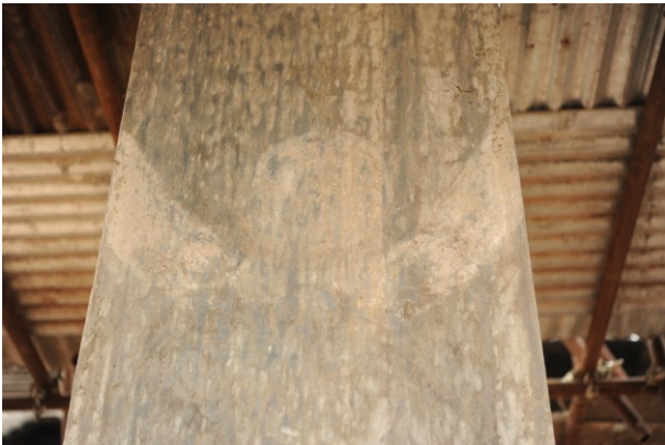
Fig. 3: Painted area at the shaft (all sides)
