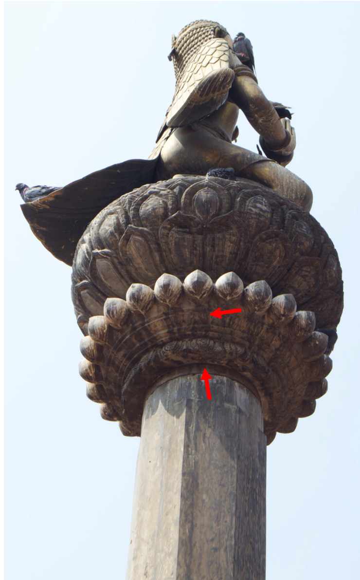
Fig. 3: Dark grey drips under the lotus seat, and rusted iron rim.
