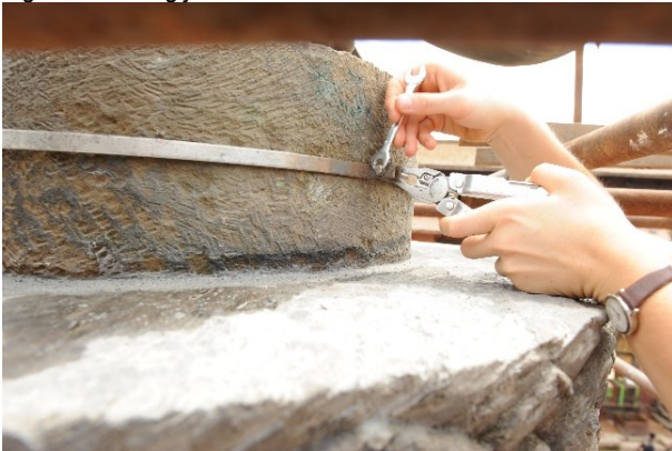
Fig. 20: Fixing and tightening the thin metal ring
