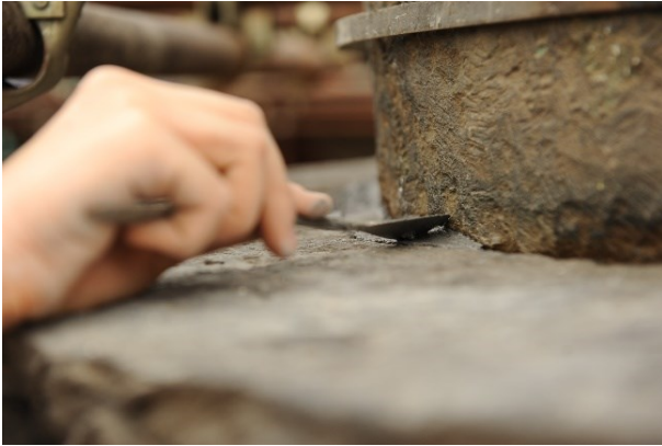
Fig. 18: Pointing joints
