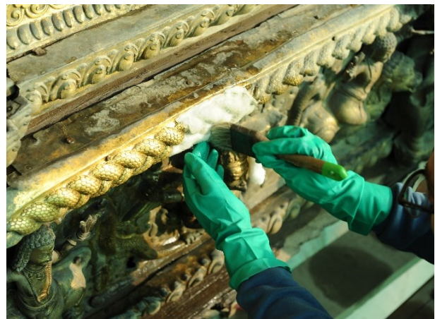
Fig. 11: Application of citric acid poultices at window
