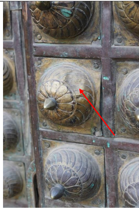
Fig. 18: Deformation (red arrow) on a knob on the right doorwing
