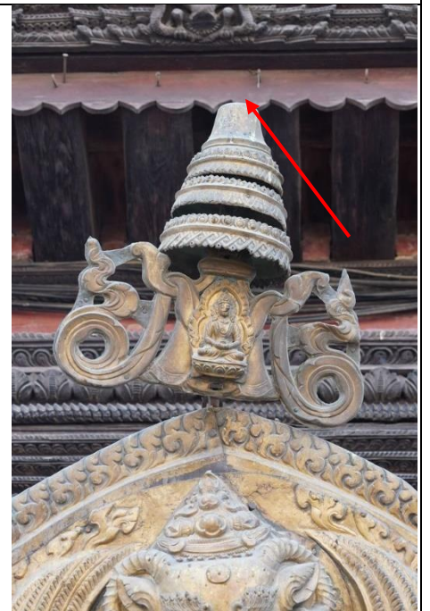
Fig. 16: 5 Missing tip on umbrella above Torana, darkening and corrosion due to soiling and bird droppings
