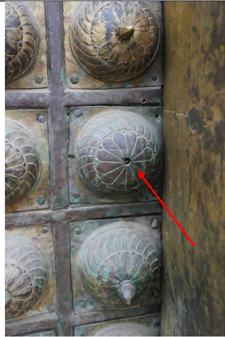
Fig. 12: Missing knob screw (red arrow) and green corrosion on the right door wing
