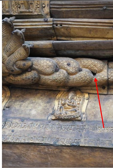
Fig. 23: Hole (red arrow) on the snake ornament, missing nail holes and secondary iron nails
