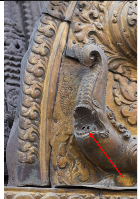
Fig. 13: Missing water spout (red arrow) on left Makara on Torana
