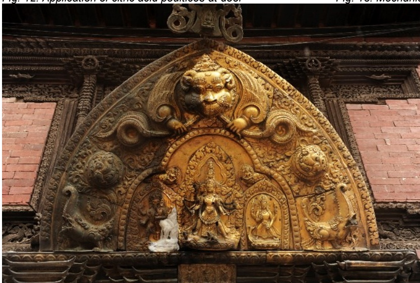
Fig. 14: Torana during cleaning
