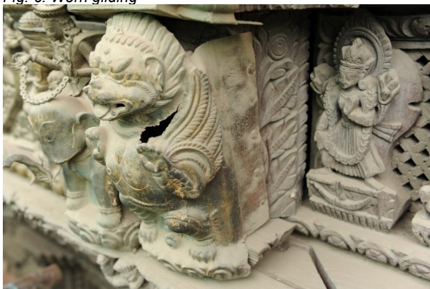
Fig. 8: Holes and corrosion on metal elements of Window
