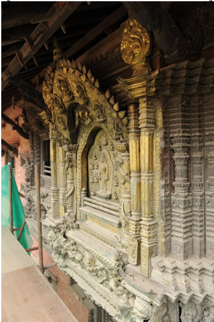
Fig. 5: Central opening of Window
