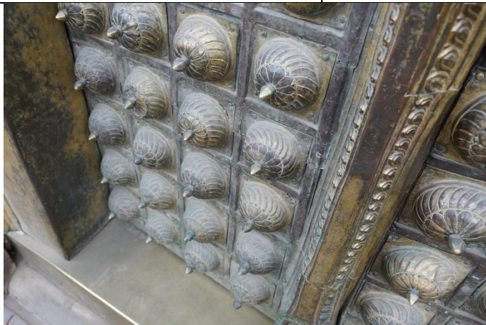
Fig. 26: Soiling and corrosion in the lower area of the doors
