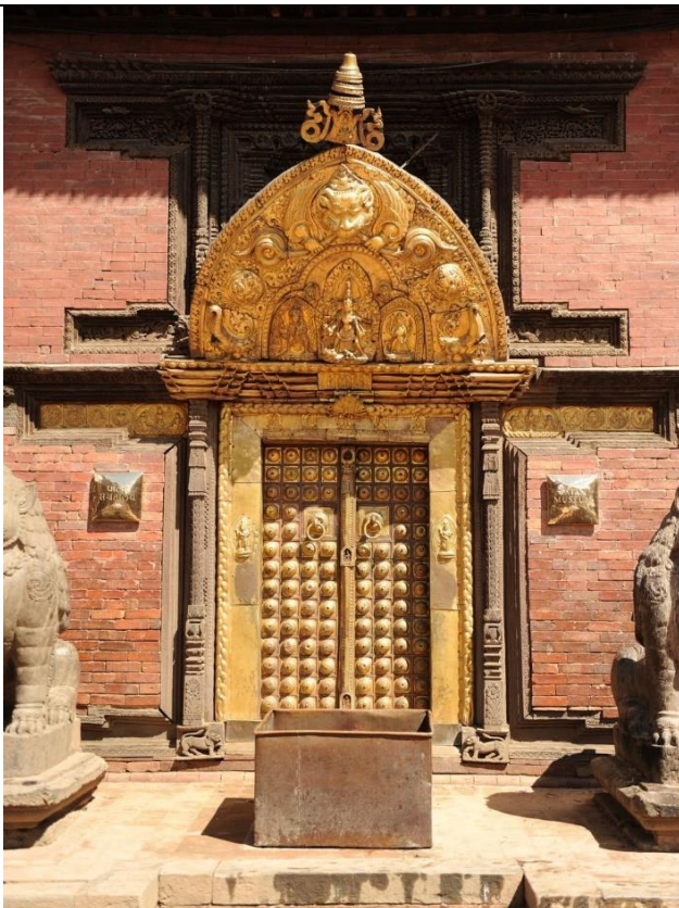
Fig. 3: Golden Door and Torana after conservation, 2018
