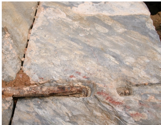
Fig. 1: Upper stone covering of Bhandarkhal Tank Pavilion Base, © loC, 2010.
