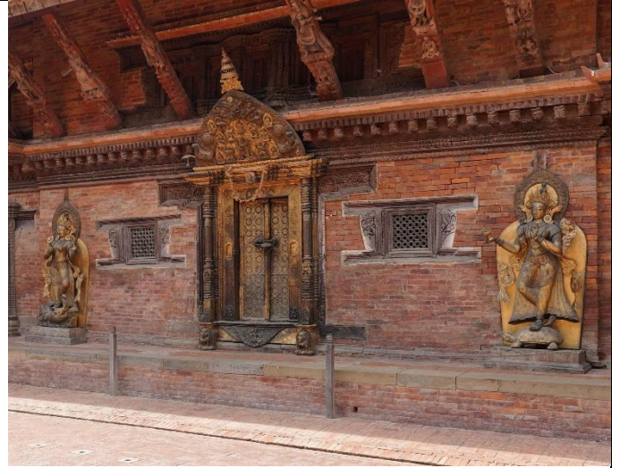
Fig. 10: Doorway ensemble in May 2024
