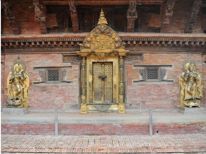
Fig. 1: Golden doorway ensemble after conservation, 2014
