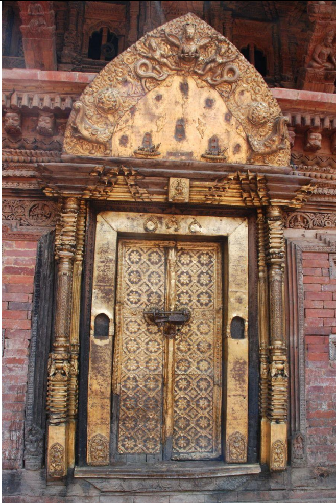
Fig. 3: Golden door and torana within the Mulchowk after conservation 2014, before final assembly
