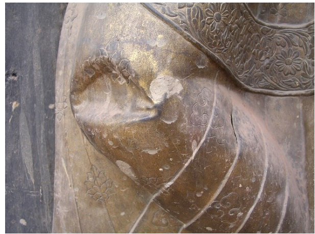
Fig. 14: Deformations and soiled surface, 2011
