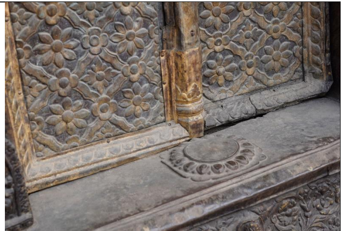
Fig. 22: Soiling and abraded, darkened surface in the lower door area
