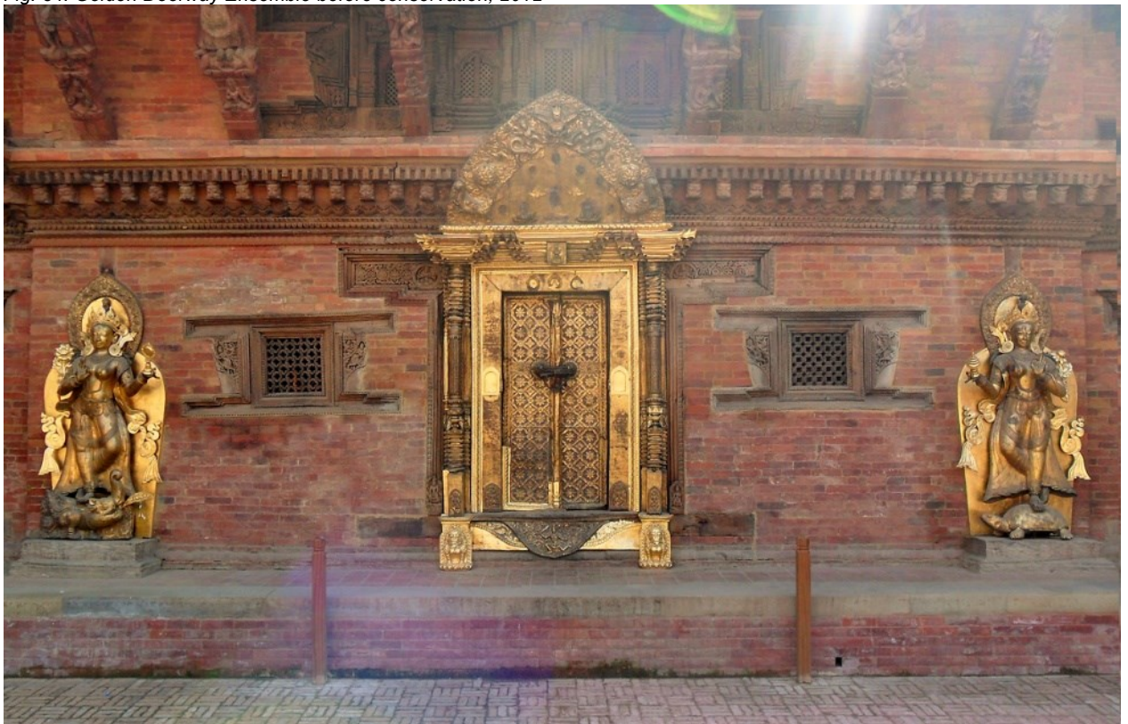
Fig. 35: Golden Doorway Ensemble after conservation, 2012
