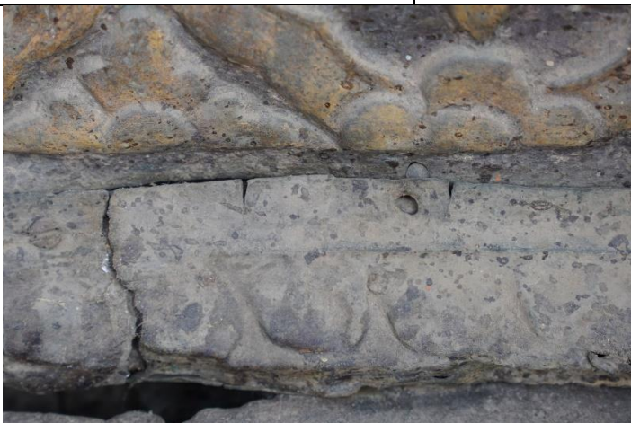
Fig. 33: Dust accumulations and blood stains on the lower door area
