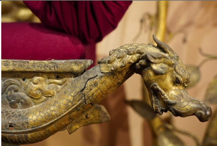
Fig. 3: Cracks in the copper sheet of the right dragon
