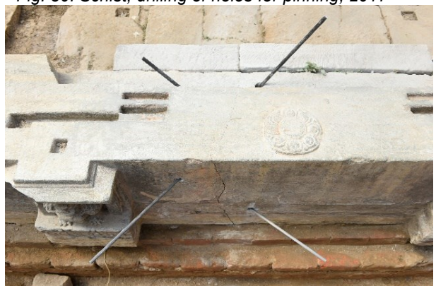
Fig. 32: Schist, reinforced threshold block (north), 2017
