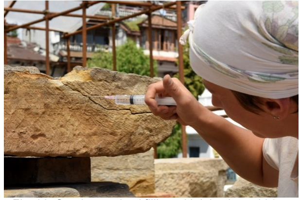
Fig. 28: Sandstone, backfilling with injections, 2017
