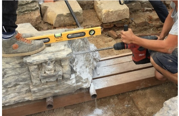
Fig. 30: Schist, drilling of holes for pinning, 2017
