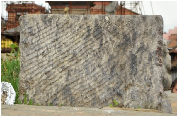
Fig. 7: Tool marks at an internal side surface, 2017
