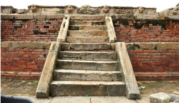
Fig. 11: Overview of stairs, 2017
