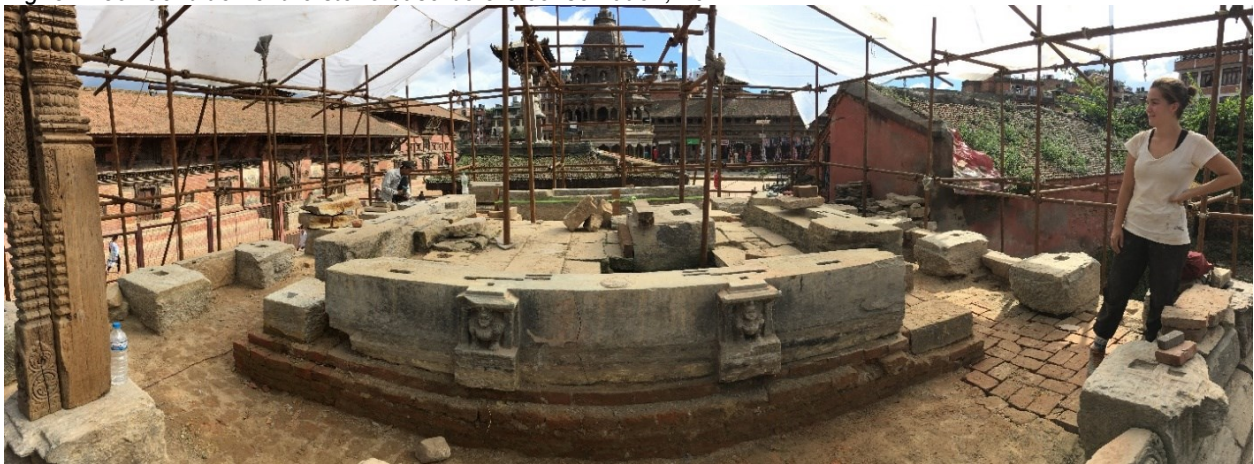
Fig. 36: Condition of the stone base during conservation, 2017
