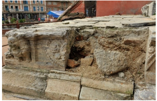
Fig. 6: Filling of the top base, 2017
