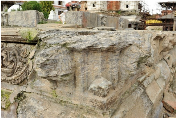
Fig. 18: Weathered cornerstone, delamination, 2017
