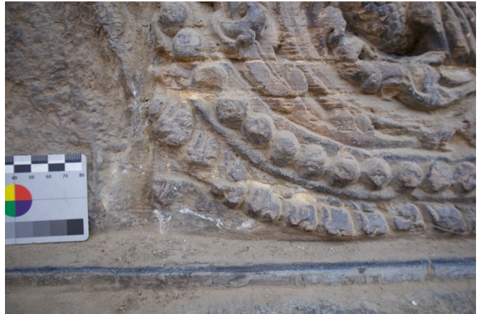
Fig. 3: Salt efflorescence.
