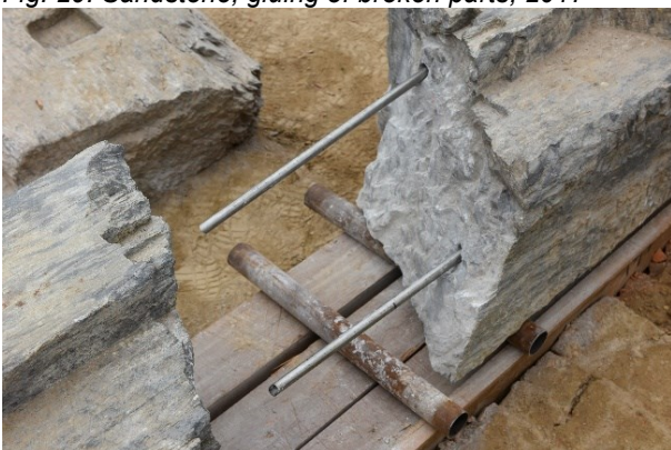
Fig. 31: Schist, pins in threshold block (south), 2017
