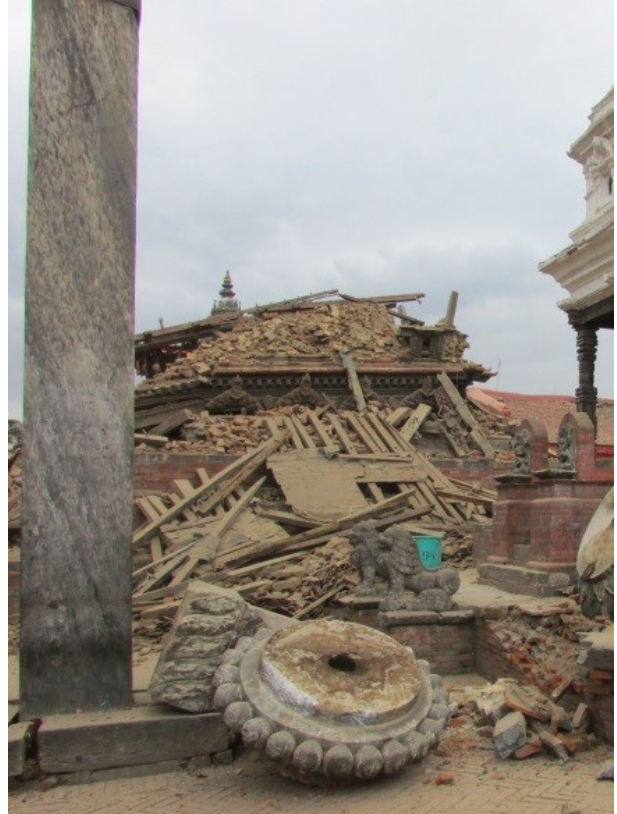
Fig. 21: Collapsed temple, 2015, © KVPT
