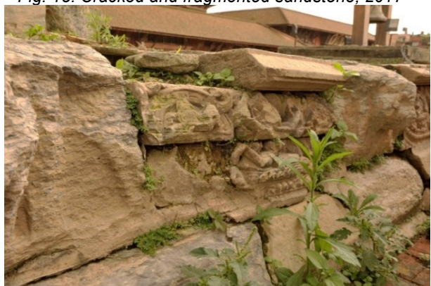
Fig. 17: Growth of higher plants within the joints, 2017
