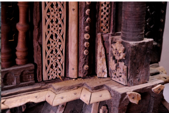
Fig. 4: Detail after conservation with brass nails, 2017
