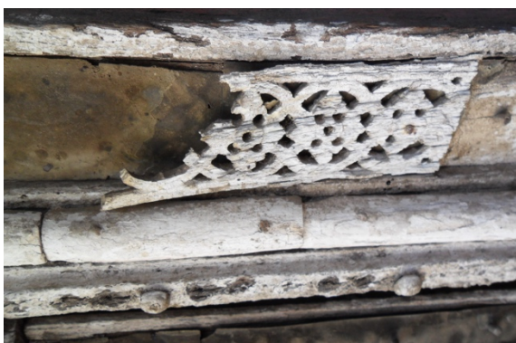
Fig. 15: Deformed, broken and brittle ivory parts, 2013
