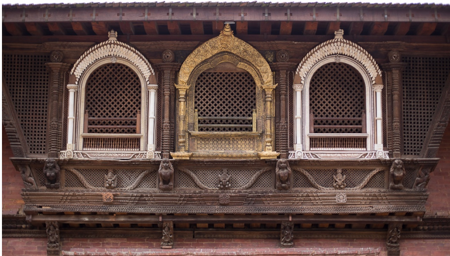
Fig. 30: Overview of the Ivory Window ensemble with reconstructed windows from the Patan Durbar Square after conservation, 2017
