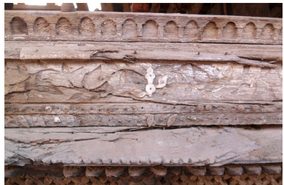
Fig. 16: Wooden support with missing ivory parts, 2013
