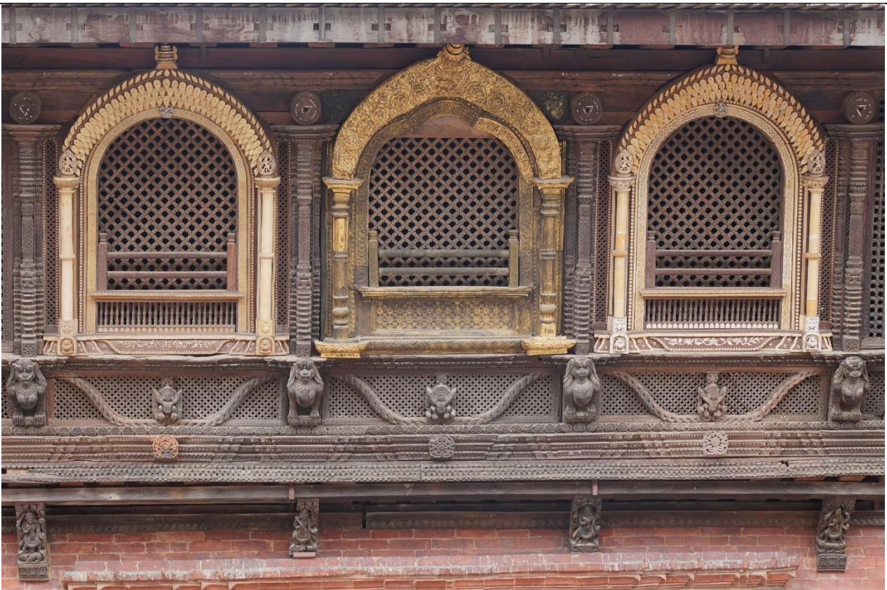
Fig. 2: Close-up of the golden window and reconstructed ivory windows on the facade of Sundari Chowk, May 2024
