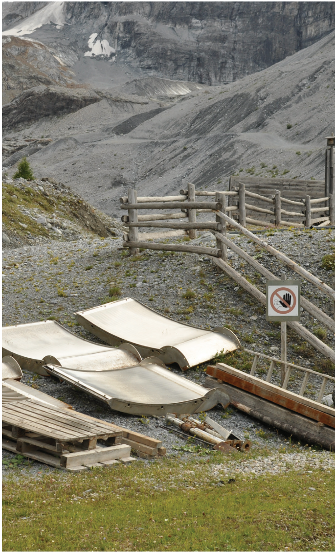
picture03_2023_bridge and dam structures at the feet of the Suldenferner glacier
