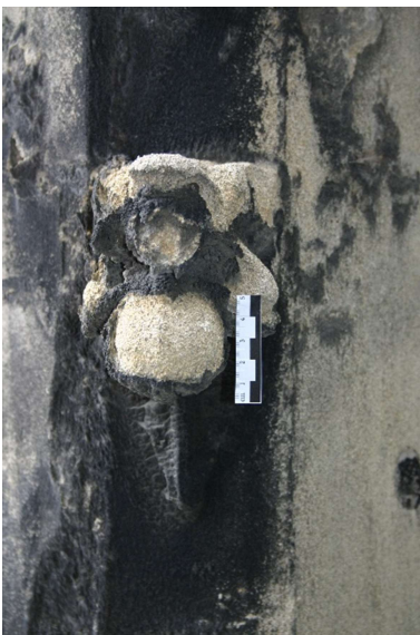
Fig. 14, 15 and 16: typical damage and decay patterns on porous limestones; f.l.t.r.: sulphation crust, salt-induced material loss and surface recession (rain exposed areas) with sulphation crust (rain protected areas)
