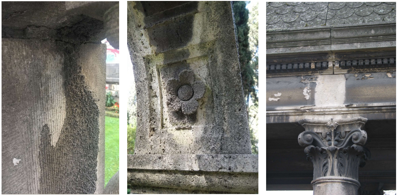
Fig. 18-20: “Black areas” or sulphation crusts, on monument surfaces in different European cities f.l.t.r.: Brussels, Rome and Vienna
