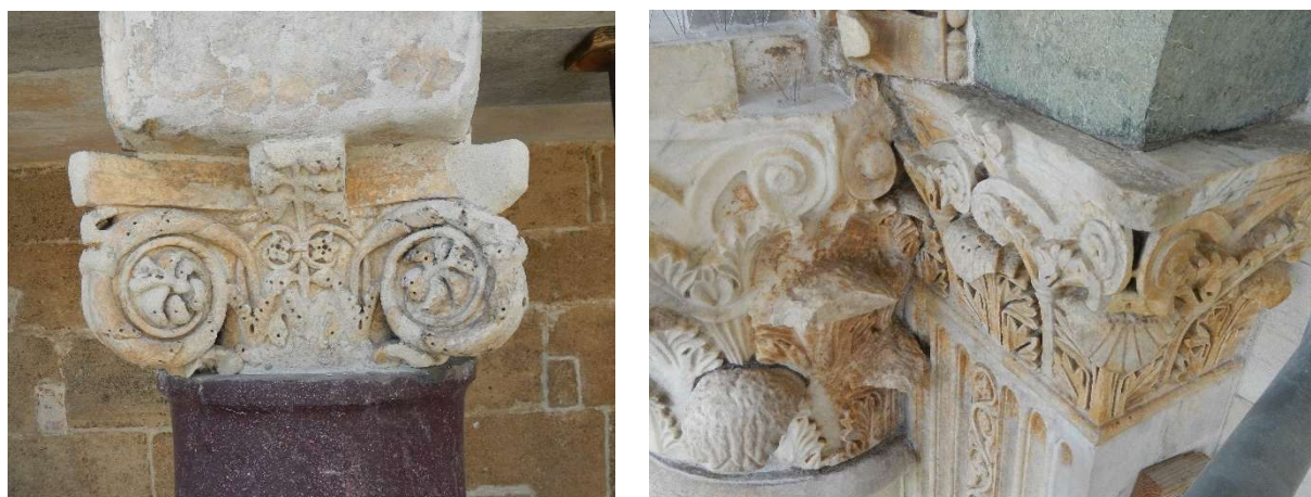
Fig. 93 and 94: Visible orange layers of natural oxalate patina on façade elements on the Cathedral of Pisa
