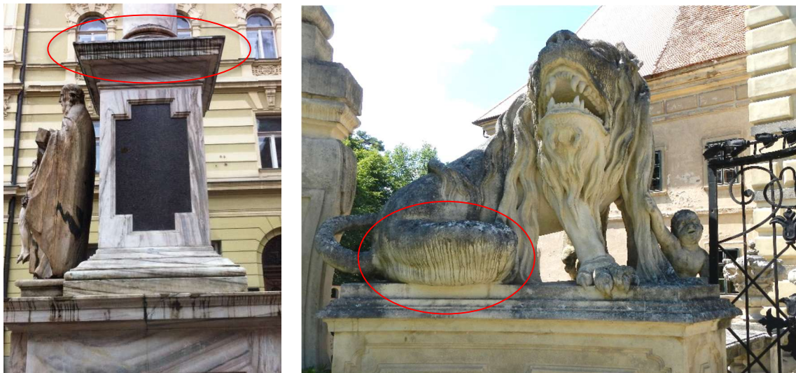
Fig. 88 and 89: Extreme soiling patterns due to a water repellent treatment documented on monuments in Austria: Klagenfurt (left) and Greillenstein (right)
