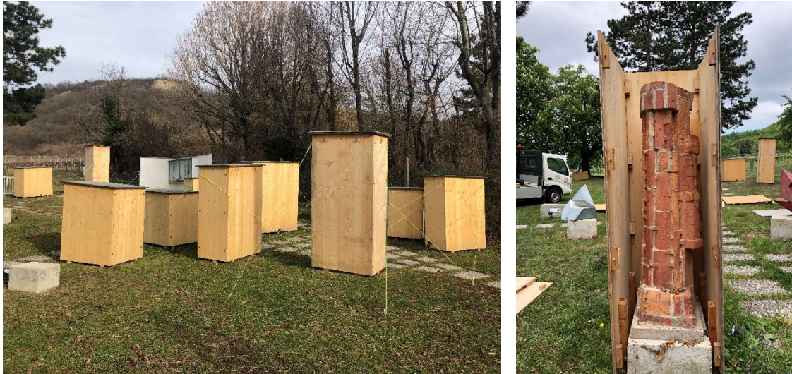
Fig 66 and 67: “Traditional” wooden winter-shelters in the museum garden of LEMU in Langenzersdorf, Lower Austria (left), one of the shelters during dismantling (right)
