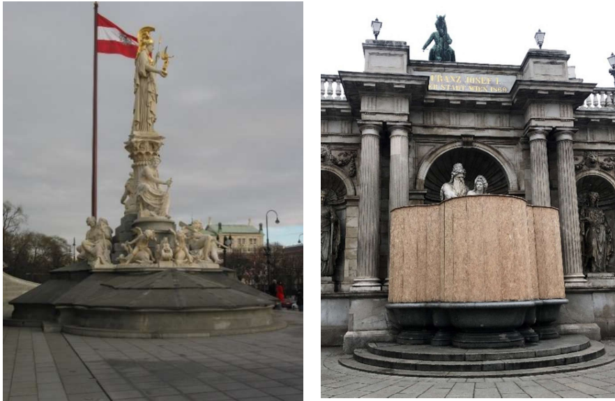
Fig. 61 and 62: Viennese fountains with winter covers for the fountain basin: Palais Athenna Fountain in front of the Austrian Parliament (left), Albrecht Fountain in front of the "Albertina" (right)
