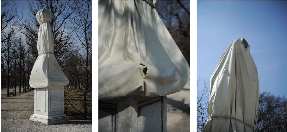
Fig. 68 – 70: soft winter-shelters in the Schönbrunn Gardens (left), prominent problems and damage (middle and right)
