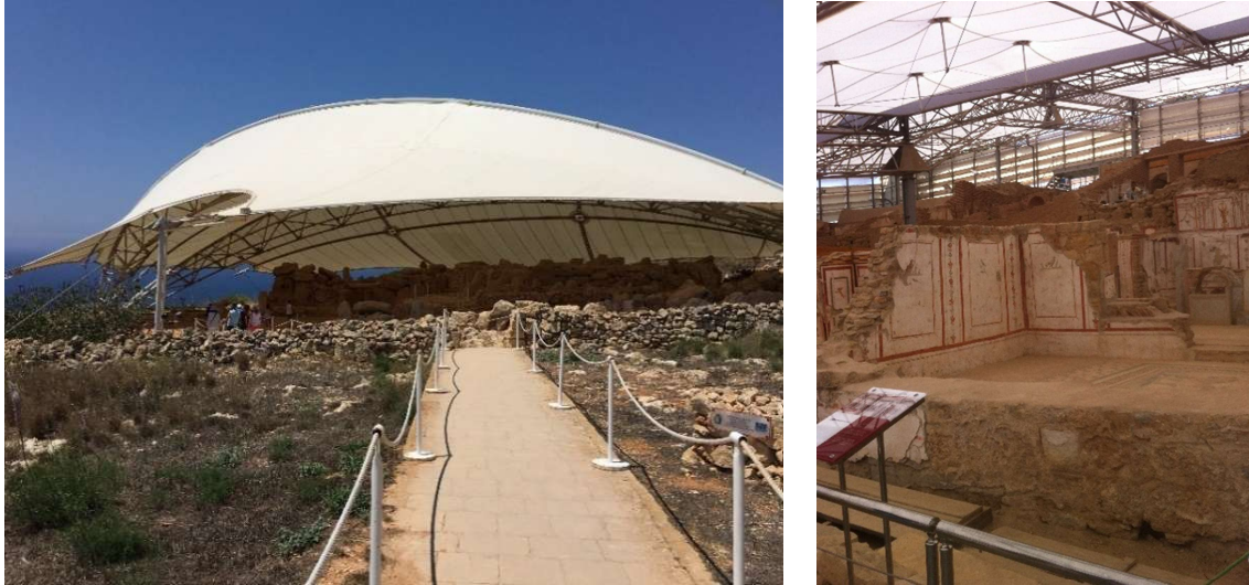
Fig. 51 and 52: permanent shelter over archaeological sites: Ħaġar Qim, Malta (left) and Slope house II, Ephesus, Turkey
