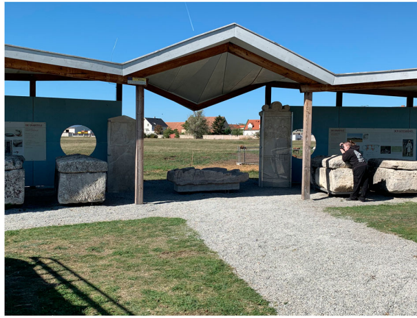
Figure 3. The permanent shelter in Leithaprodersdorf protects Roman sarcophagi and gravestones.
