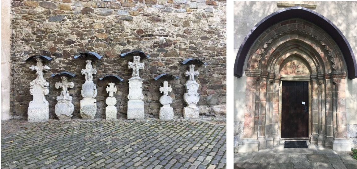
Fig. 48 and 49: permanent roofs as protection: left: historic roofs over gravestones on a church façade in Eggenburg, Lower Austria; right: a contemporary roof over a stone portal, St. Pantaleon-Erla, Lower Austria
