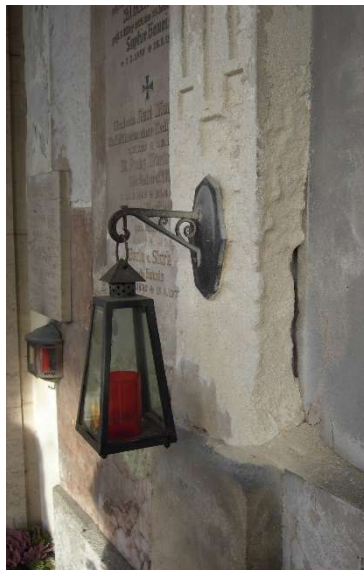
Fig. 14, 15 and 16: typical damage and decay patterns on porous limestones; f.l.t.r.: sulphation crust, salt-induced material loss and surface recession (rain exposed areas) with sulphation crust (rain protected areas)
