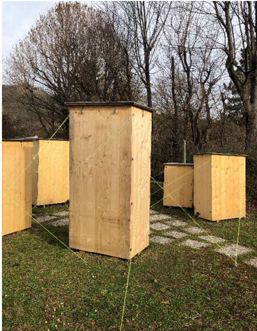
Fig. 77: Wooden shelters stabilised by tension ropes
