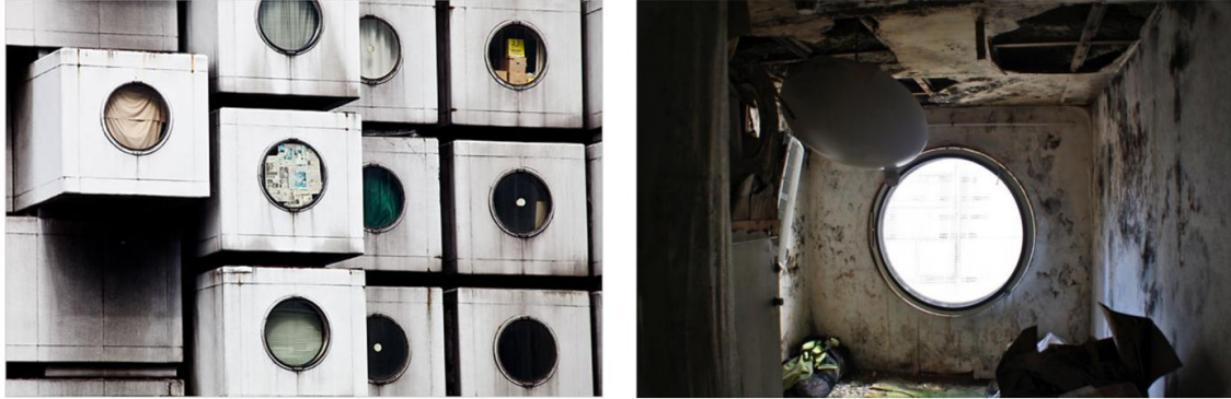
Figure 2-15: the lack of maintenance in the Nakagin tower, Source of left photo:(O'Connell, 2009), right photo:(Soares and Magalhães, 2014)
