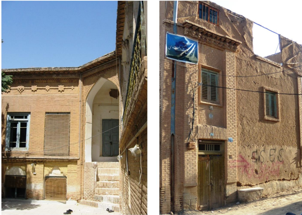
Figure 2-33: left- simple mat curtain on the main façade of the Kian house in Sabzevar (Qajar) Right- shutter windows on a west facing façade in a Pahlavi house in Sabzevar
