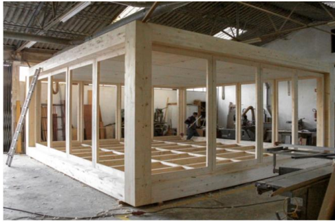
Prefabricated modular construction
