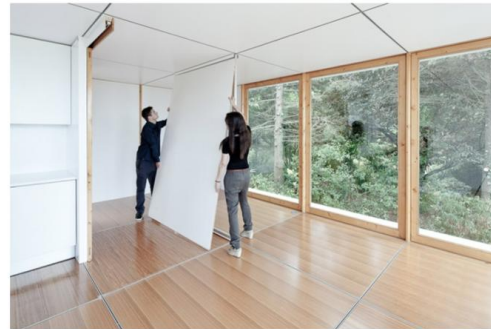
Placing modular wall in grids of rails
