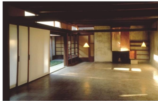
2- Modular Structure and sliding panels in Schindler House, West Hollywood, US, 1921-22
