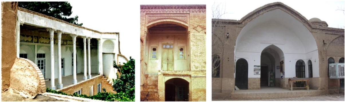
Figure 6-12: left: pillared portico (veranda) of Baqani house (Kermani-Moqaddam, 2002b), center: simple Eivan (flat roof) of Cheshomi house, source: the local archives of ICHTO in Sabzevar, right: vaulted Eivan of The Mashhadi house (Estaji, 2010)
