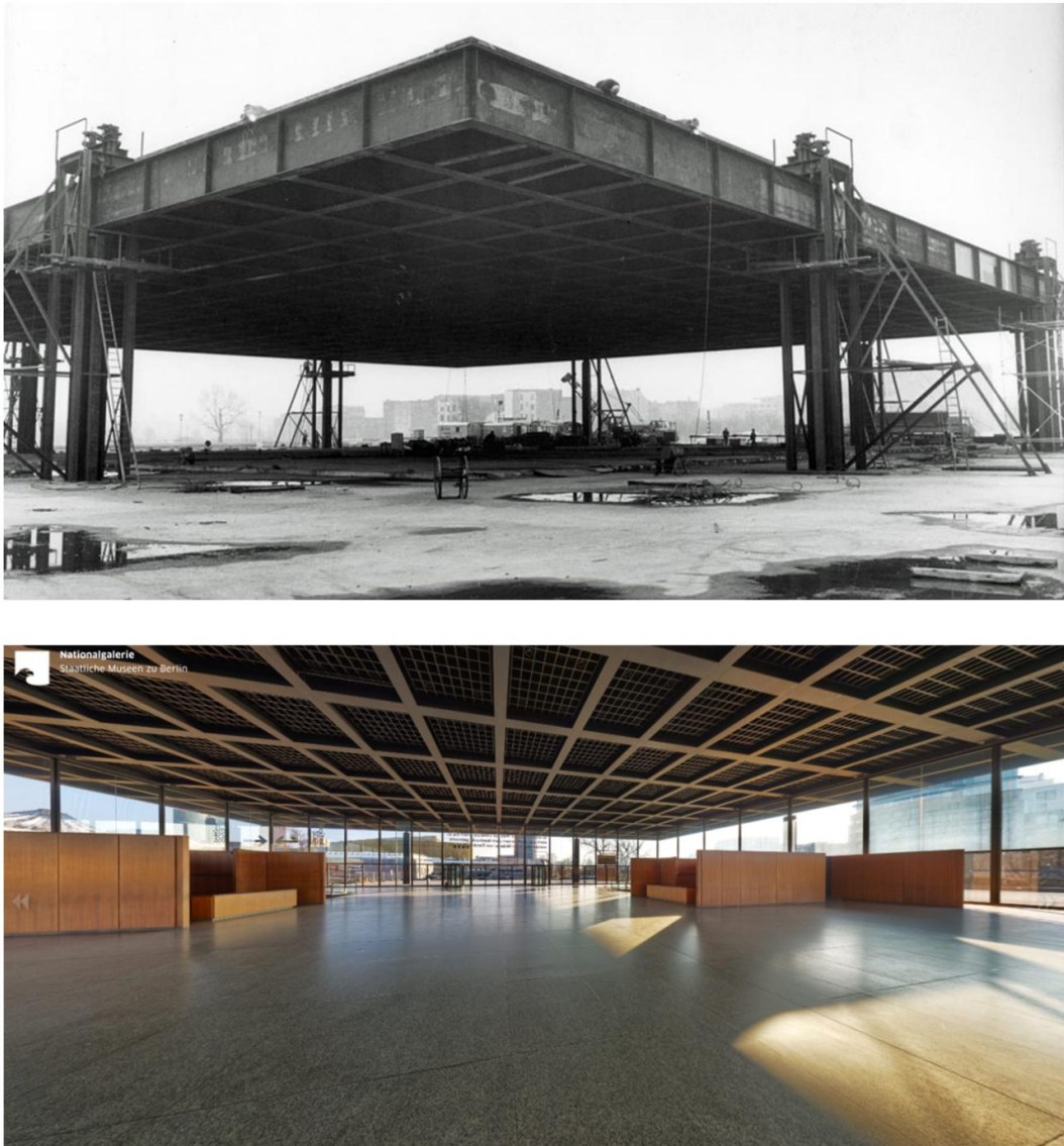
Figure 2-20: top- The steel roof structure of the new National Gallery Berlin, taken in 1967©SMB, Zentralarchiv (Preussischer Kulturbesitz, 2016), bottom: the interior space of the gallery (Neue Nationalgalerie, 2016)
