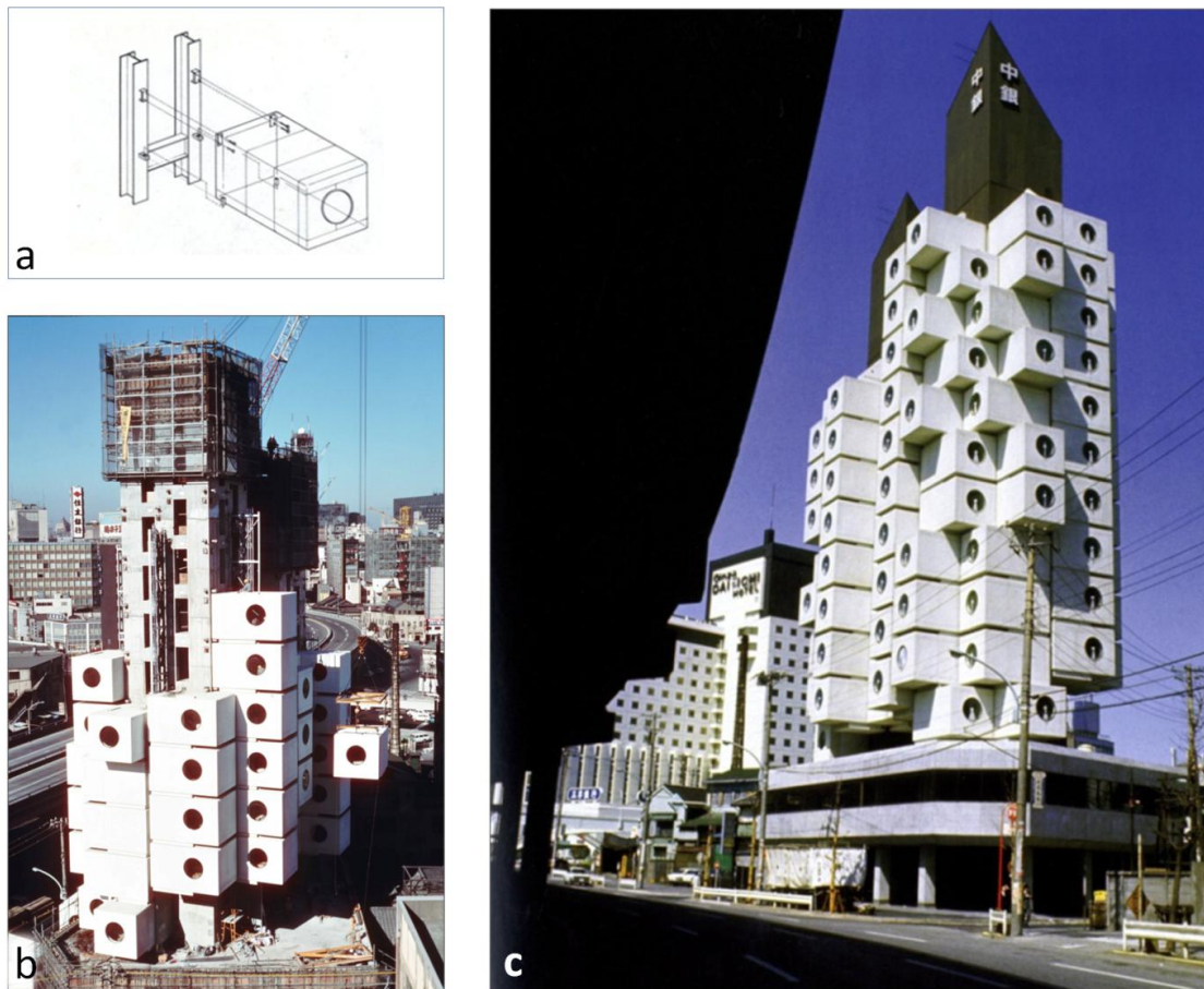
Figure 2-14: a- detail of joining a capsule to the shaft (Kurokawa, 1977, p. 108), b- assembly process (Bergdoll et al., 2008, p. 145) c- street view of Nakagin tower (Kurokawa, 2015)
